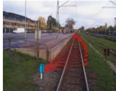
Alam system for people falling on the rail tracks in a station
